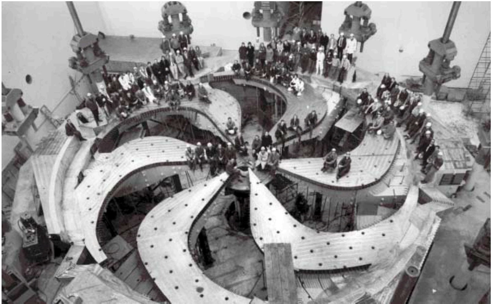
Lower half of the Main Magnet poles
